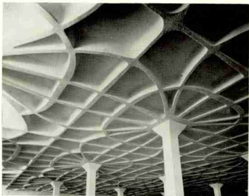
Constructional and static solution - the ribs follow the lines of principal bending moments. The elegance of these lines is not due to the merit of the designer but is a merit of the structure itself.
