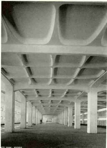
Italian State Tobacco Factory (1949). Movable precast concrete forms.
