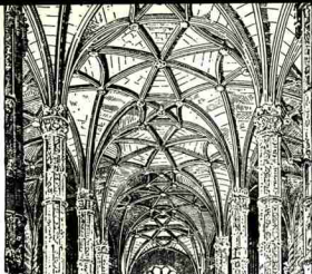
Figure 32. Star vaults in the central nave of the Church of Jeronimus at Belem near Lisbon, interpenetrating with those of the lateral naves. From the joining disappear the arches of the peripheral supports, substituted by fusiform vaults. This is a celebrated major work of Portuguese Eusebian art, from the king Emanuele I (1495-1521).
