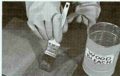
Figure 2. Use rubber gloves while applying bleach to the wood surface.
