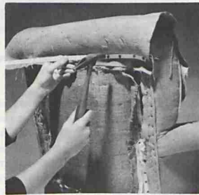
Fig. 53—Blind tacking outside back at top.
