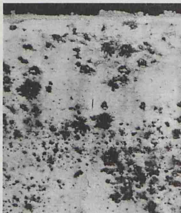
Diffused discoloration caused by rain and dew penetrating a thin porous paint film.
