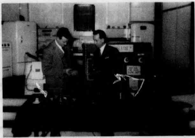
Above is pictured Mr. W. J. Rideout examining an entrance switch while Mr. Paul T. Tysinger looks on.
