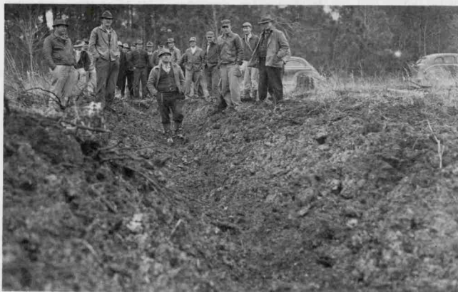
B. "Dynamite supplants labor in ditching," read the Beaufort County headlines in 1946. Howard Ellis is second from left.
