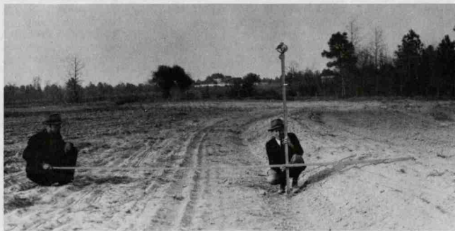
Fig. 17. H.M. Ellis holds the rod indicating the depth of a completed broad-base Mangum Terrace on the William Collins farm, Nash County, in 1942.
