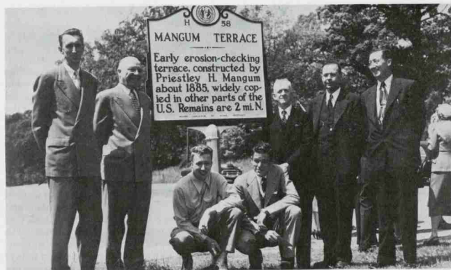
Fig. 16. The above picture was taken at the erection of the historical marker at the site of the first Mangum Terrace in the United States. Standing (left to right) are G.W. Giles; J.H. Hilton, Dean of Agriculture; Priestley H. Mangum, III; D.S. Weaver, Director of Extension; and H.M. Ellis. Kneeling are F.Z. Blevins (left) and B.S. Sutton representing the ASAE Student Club.
