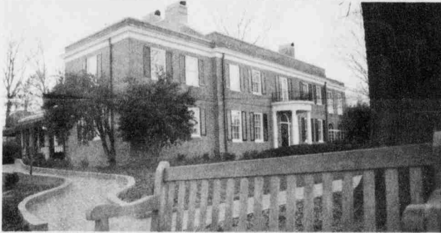
The Chancellor's house recently received $171,900 in renovations.
