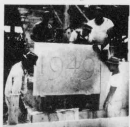
Workers set the cornerstone of Reynolds in place in 1949.
