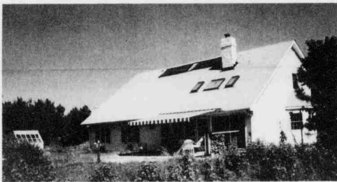
Thomas Wentworth's solar house looks like a regular house.
