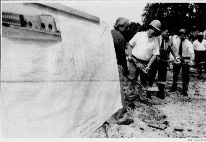
A group of campus leaders and local contractors throw back the first shovelfuls of dirt at the future site of NCSU's Student Health Center.
