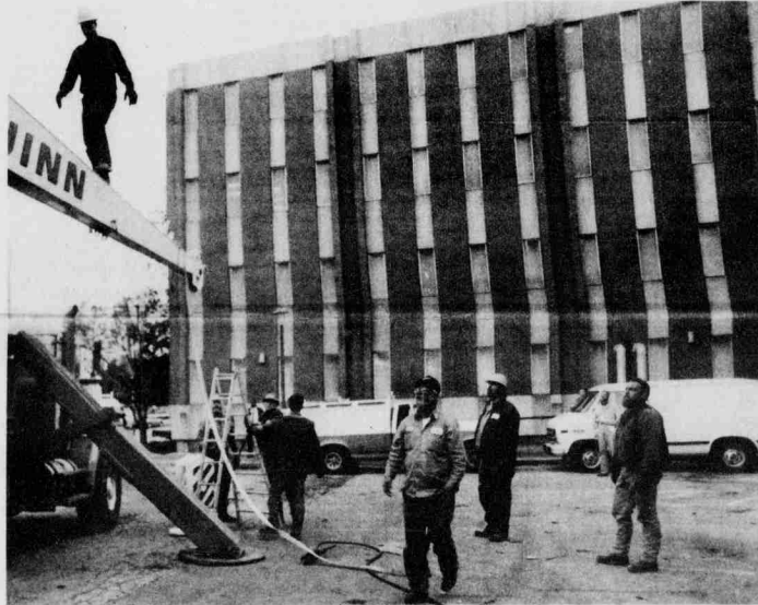
A worker (left) carefully paces across some heavy machinery outside of Gardner Hall Tuesday. The construction crew shown is replacing the cooling system of Gardner Hall.
