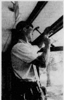
Brett Zick of Cornerstone Construction Company helps repair a fire exit at the Sigma Alpha Epsilon house.
