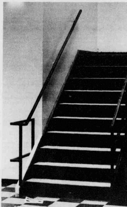
The stairs at the Sigma Alpha Mu fraternity house do not lead directly to the exit, which is a fire code violation.
