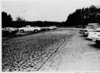
Cracks have formed in the part of the Kmart parking lot where Wolfline buses pick up park-and-ride N.C. State students.
