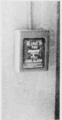
Glass-cased fire alarms like this one have tempted pranksters this summer.
