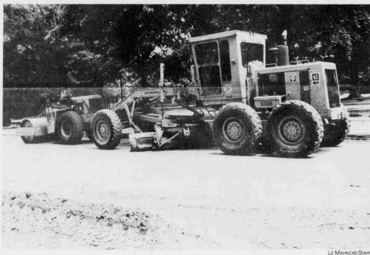
Students may have noticed the construction that seems widespread across campus. The repairs are a part of an effort to get ahead of some troublespots before traffic is too heavy in the fall and spring.
