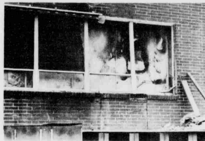
A view of the damage caused by a morning fire at the Plasma Center on Hillsborough St. The fire caused only minimal damage.
