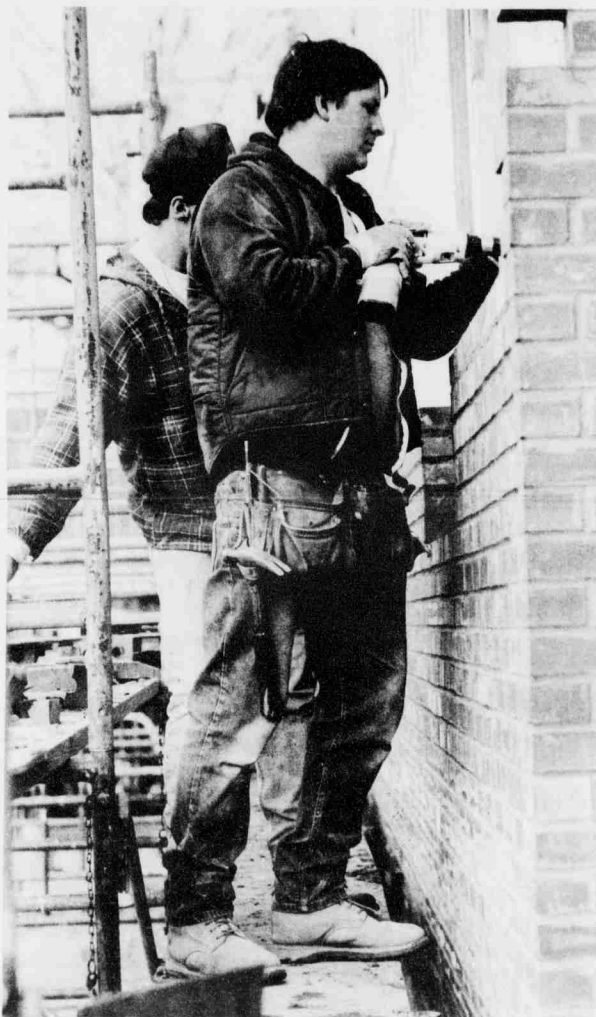
A Polovick Construction employee works on expanding Polk Hall. Polovick plans to have the extension completed within two weeks, weather permitting. Other campus construction includes turning bricks over to prevent them from decaying. Yes, really.
