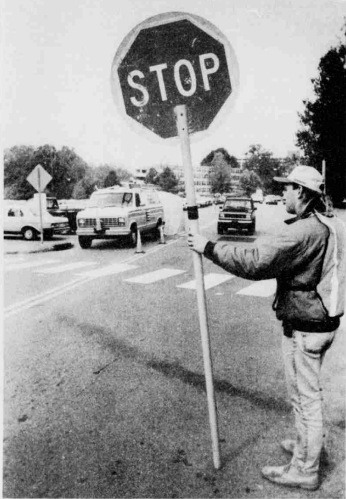
Alan Murphy of Southern Bell directs traffic as fellow workers repair NCSU's phone wires under ground.
