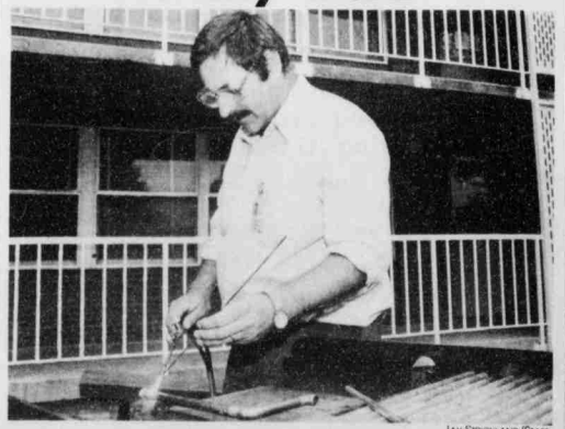
Bobby Norris, a 12-year employee of the Physical Plant, fixes a leak in a steam pipe at Bragaw Residence Hall Tuesday.
