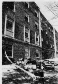
Fire debris was piled next to dorm.
