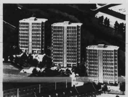
Construction on Bowen, Metcalf, and Carroll dormitories will begin in two to three weeks.
