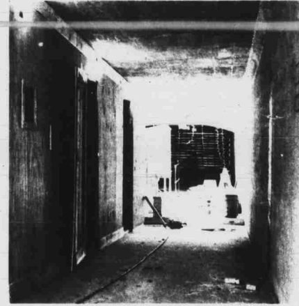
The tunnel leading to the Harrison Hall area is now closed and used for tool storage instead of providing convenient access to classroom buildings. (Photo by Holcombe)
