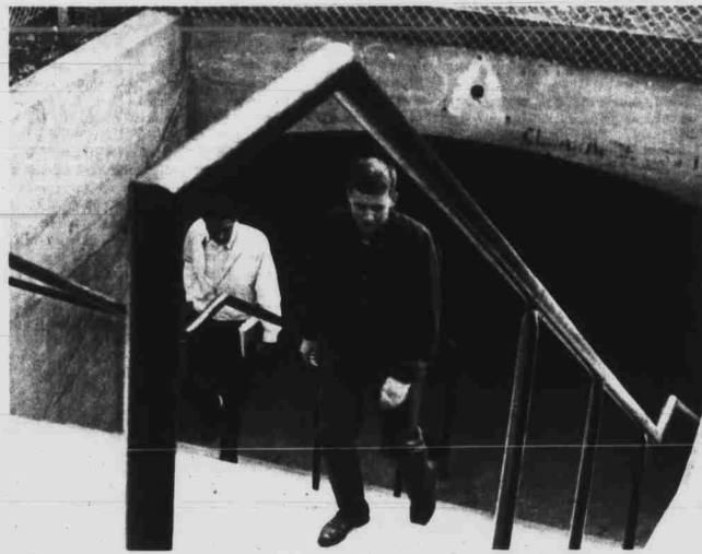
A stairway terminated on Yarborough Drive has been constructed by the Physical Plant in order to reopen the tunnel formerly connecting the Supply Store Mall and the Harrelson Hall area.
