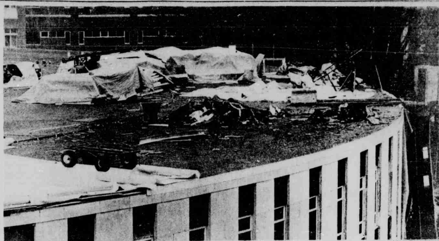
Is the sky falling or is the roof just caving in? Neither. It's just a renovation project for the roof of Harrelson Hall. Mark RUSH/STAFF
