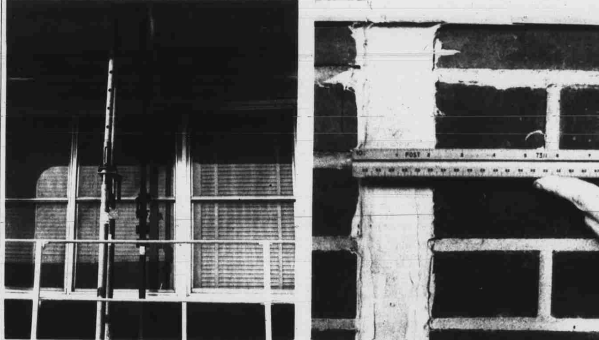
Although there is not much chance that Lee Dormitory will fall in the immediate future, there is definite indication of trouble. The cracks which have appeared and the jacks which have been erected have resulted in considerable interest on behalf of the students.
