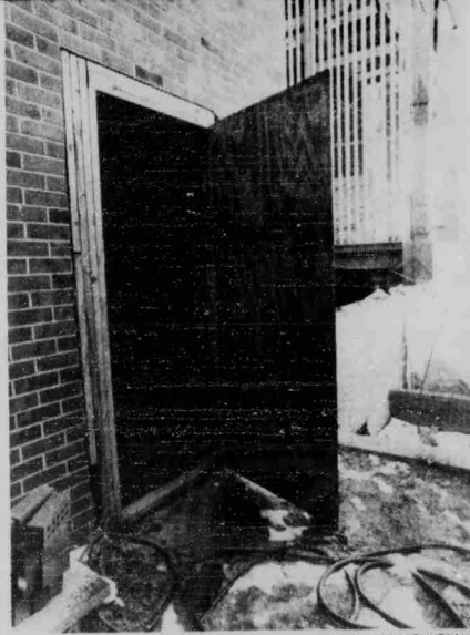
Unlocked doors such as this one can account for the fact that D.H. Hill Library has lost 3.4 percent of their holdings since 1980.
