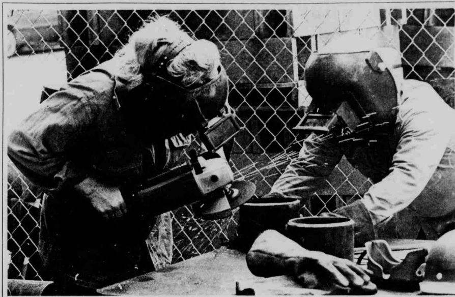
many construction workers on campus grind plumbing fittings for the additions being made to Withers Hall.
