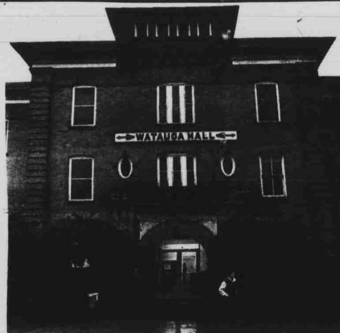
Watauga Hall has gone through some extensive changes since it was built. It is shown here as the home of the Campus Construction and Planning headquarters.
