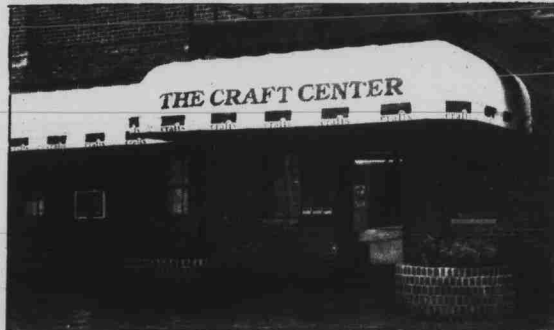
lower level Thompson building, across from parking deck; south campus
