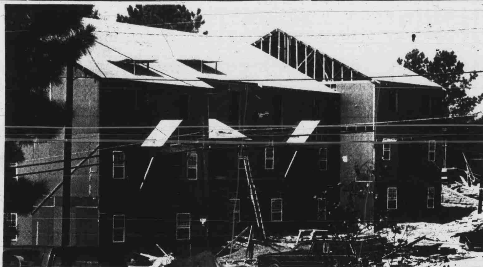
Construction continues on the 120 unit Avery Close condominiums located on Avent Ferry Road at Varsity Drive. Construction on the development,
