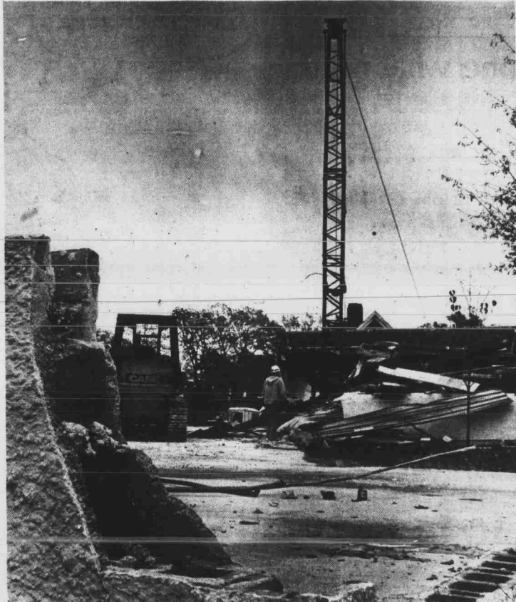
Destruction has begun on the Hillsborough Square buildings. State changed its plans to renovate the buildings. It now plans to build new buildings using similar architectural designs.
