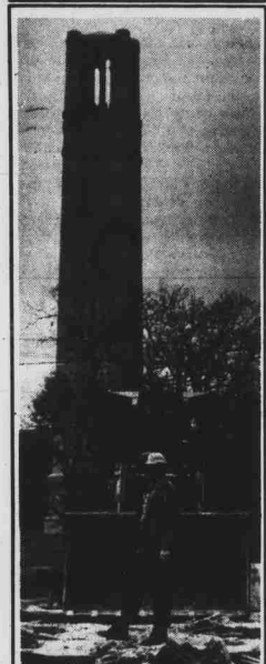
Staff photo by Clayton Brinkley Hillsborough square renovation plans have been changed, and the University is now in the process of demolishing all the buildings with an 'unsafe' status. See Wednesday's Technician for details.
