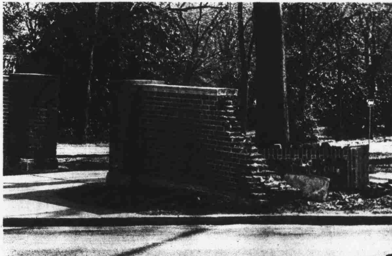
The brick wall that was damaged before spring break by a truck is now scheduled for repair by the Physical Plant. The delay was caused by an insurance settlement.
