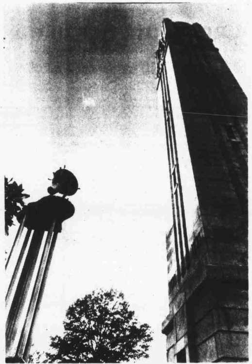
Vandals partially destroyed one of the lamps surrounding the bell tower (above left). The repairs for the lights that were destroyed (above right) is estimated at over $2,000.
