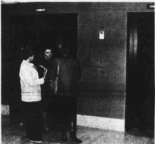
Elevator breakdown in the Student Center is not only an inconvenience but may affect revenue due to students' inability to take the elevators to the fourth-floor Walnut Room. Staff photo by Clayton Brinkley
