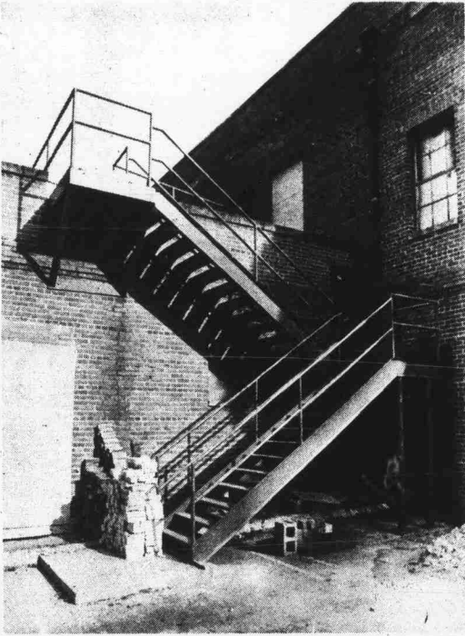
State's rifle range was closed by the Division of Student Affairs last spring after an inspection revealed unsafe conditions.
