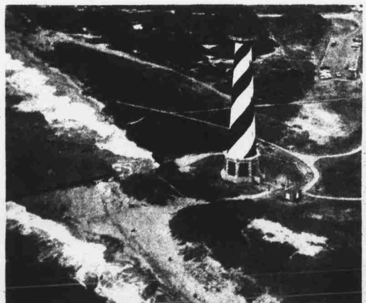
Sand washed over from the beach almost reaches the door at the base of the Cape Hatteras Lighthouse.
