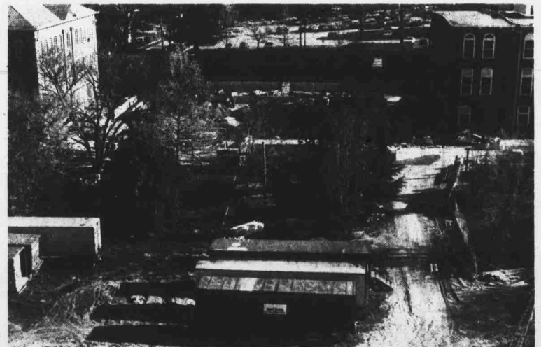
The foundation for the Link Building between Tompkins and Winston halls is 85 percent finished. Completion of the building will be delayed at least one month, due to weather conditions. (Staff photo by Simon Griffiths)
