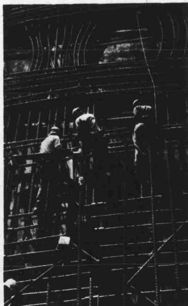
Workers place reinforcement bars around the steel liner of the first Harris reactor. As many as 10 layers of the steel bars will be used in the four and a half foot thick concrete walls.
