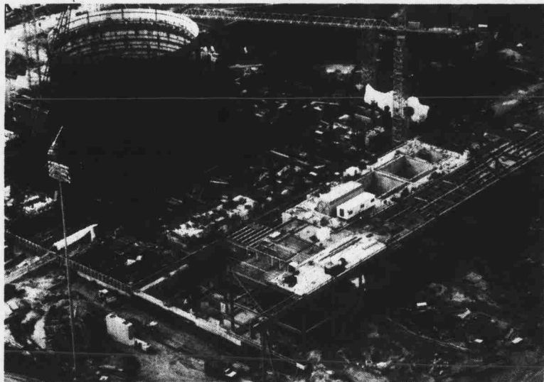
An aerial view of Shearon Harris Nuclear Power Plant Unit One under construction.
