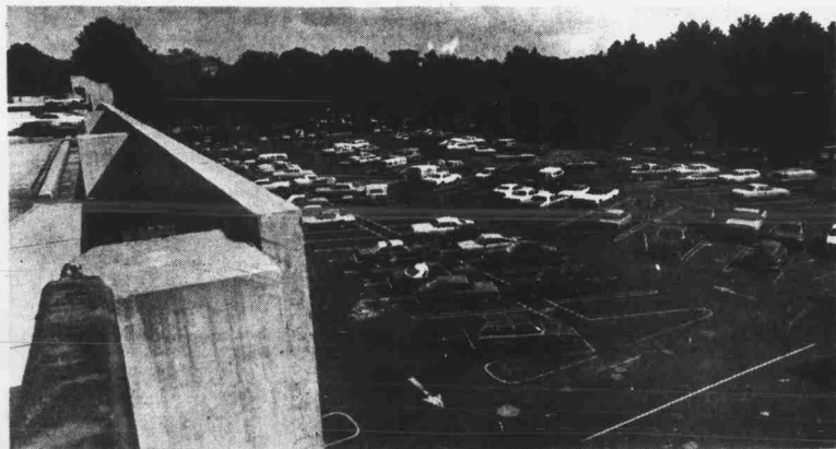
While this parking lot rests before the morning onslaught of traffic, the construction of a new parking deck is being recommended by the Transportation Committee. (Staff photo by Steve Wilson)
