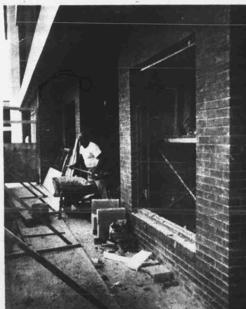
Construction and installation of two 24-hour banking machines in the Student Center should be completed by mid-October. (Staff photo by William Proctor)
