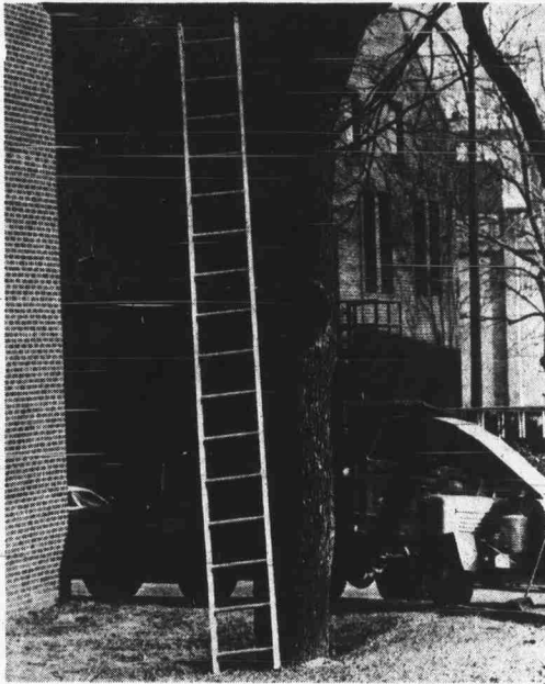
Staff photo by Wayne Bloom Ice damage You could draw a lot of conclusions from this one. If there was a fire truck we'd guess there was a cat in a tree. More likely, the recent ice storms have done their share of damage and the repairs are going on.
