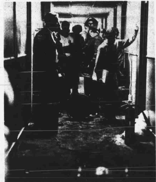
An undetermined amount of damage was done to 230 Tucker in a Sunday fire.
