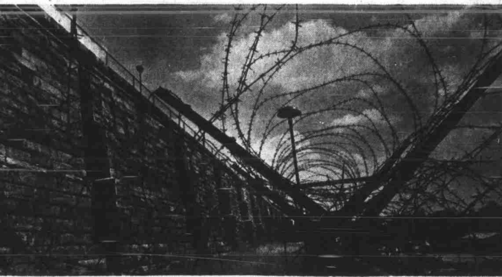
With the existing Doak Field Fence proving to be an inadequate barrier to various and sundry commonplace students, Director of Athletics Willis Casey has contracted with Central Prison to lease their fortress which is being presently transferred to Doak Field. "We'll keep the scum out at any cost," Casey said quoting a round figure of $10,000 a day for the new erection which will be covered by a rise in student fees.
