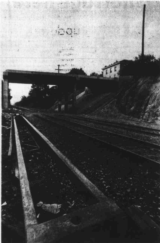
State has agreed to pay for some of the pavement on the new Pullen Bridge because the paving had to be done solely for State's benefit. Also, State will pay for the water tubing to be hung under the bridge, in order to connect the University's fire hydrant system.
