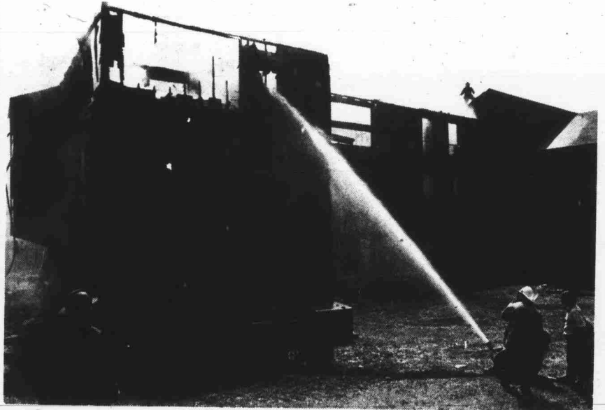
The result: a building somewhere else may burn almost beyond salvaging, like this one at a local apartment complex did.
