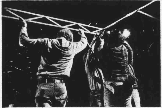
Reconstruction begins on Carmichael Auditorium after Saturday night's concert brought down the house.
