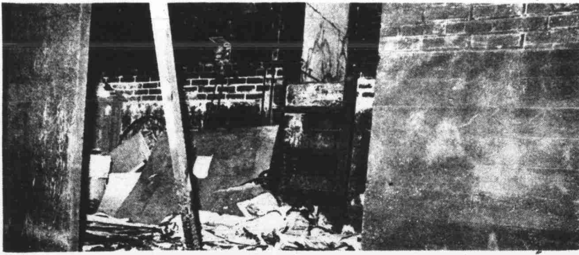
An early morning fire did between $20,000 and $25,000 damage to the Studio One theatre last Wednesday morning. Raleigh Fire Department officials suspected a carelessly thrown cigarette caused the fire. Arson was not suspected and no one was injured in the blaze. Theatre officials said they expect the theatre to be closed from a week to ten days.
