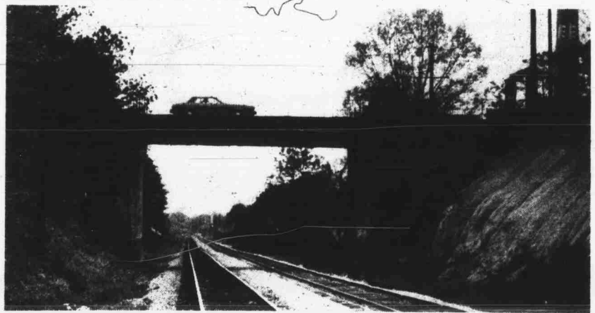
The city of Raleigh has recently decided to tear down the Pullen Bridge due to faulty architectural construction. Officials estimate that it will take nearly nine months to tear down the present structure and build a new one.
